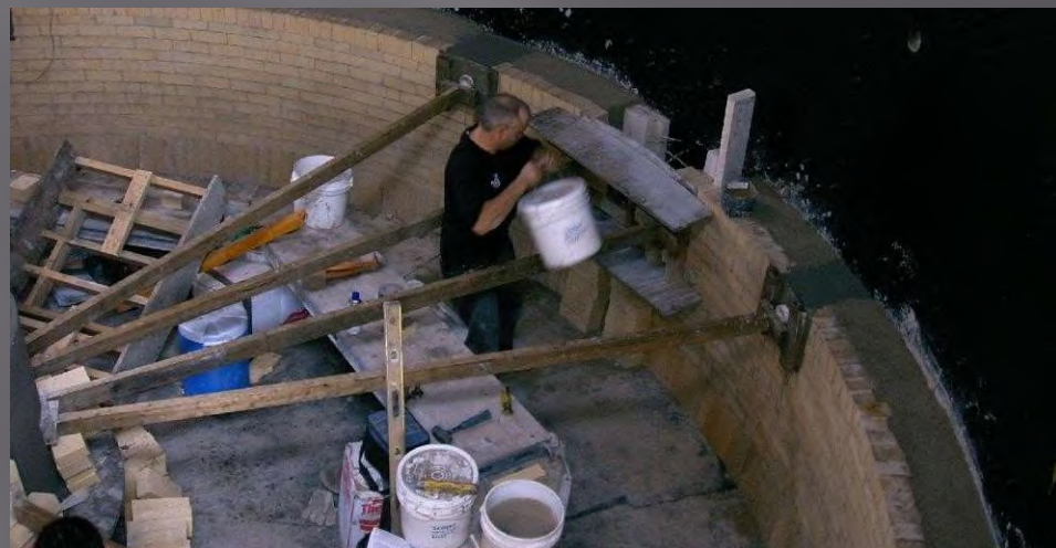
A crew installing a new furnace wall lining and hearth. In this photo they are pouring a refractory burnertile.
