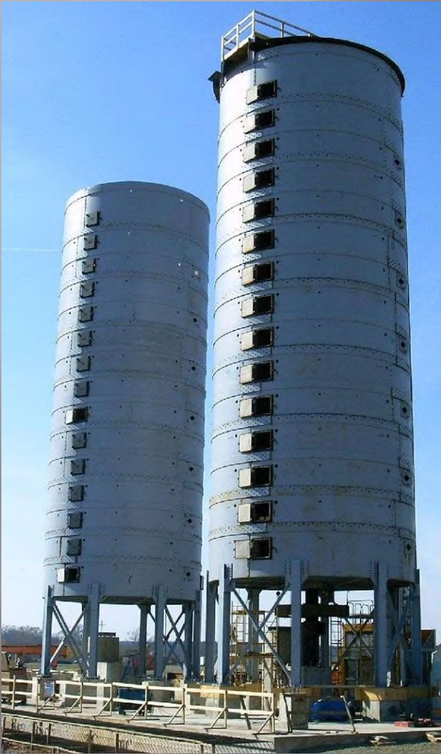
Two large MHFs under construction
